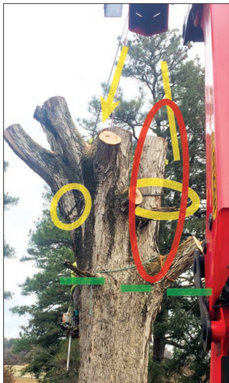
Photo 3: The yellow highlights are the lifting bridle. The green highlights show the location of the cut.
